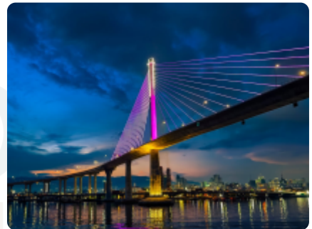
Cebu City, CLELEX bridge illuminated at night, reflecting vibrant colors over the water.
