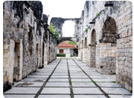
Cuartel Baluarte Ruins in Oslob, Cebu, Philippines
