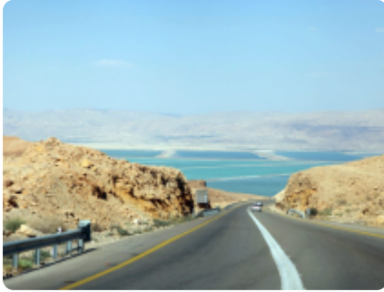
Highway to Sinai, Road 90-Arava valley, Israel
