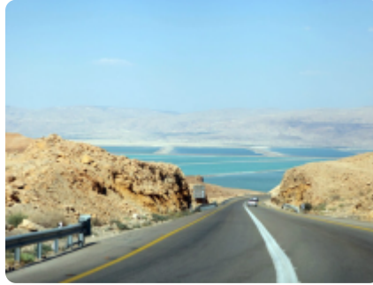
Highway to Sinai, Road 90-Arava valley, Israel
