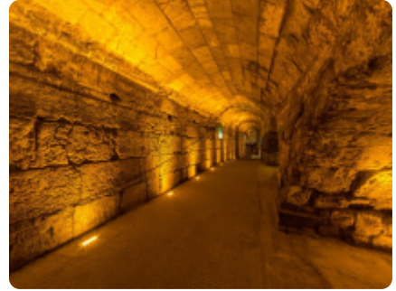
Western Wall Tunnels, Jerusalem, Israel
