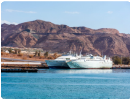
Aqaba ferry terminal, Aqaba, Jordan
