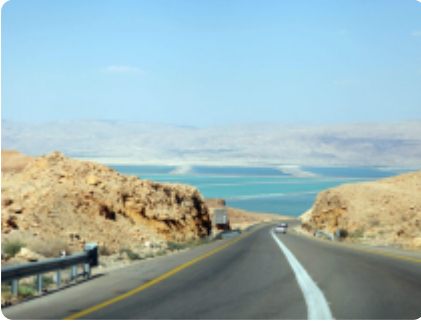
Highway to Sinai, Road 90-Arava valley, Israel
