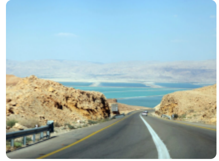
Highway to Sinai, Road 90-Arava valley, Israel
