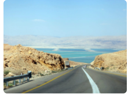
Highway to Sinai, Road 90-Arava valley, Israel
