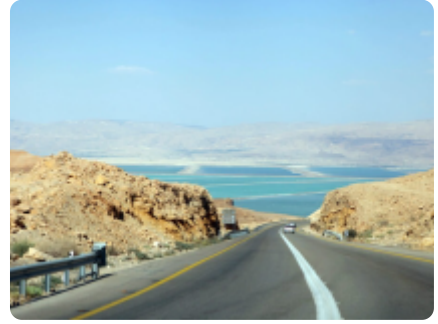
Highway to Sinai, Road 90-Arava valley, Israel
