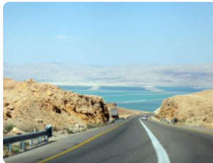
Highway to Sinai, Road 90-Arava valley, Israel
