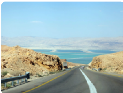
Highway to Sinai, Road 90-Arava valley, Israel
